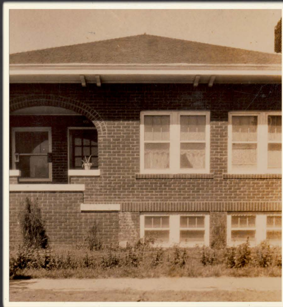
The Correll home at 506 Colgate completed in 1928. This is a "True" brick home constructed of two layers of brick. Notice the original front stairs with steps on either side. It was suggested they were changed because in this configuration rain water was channeled directly to the front basement windows.
