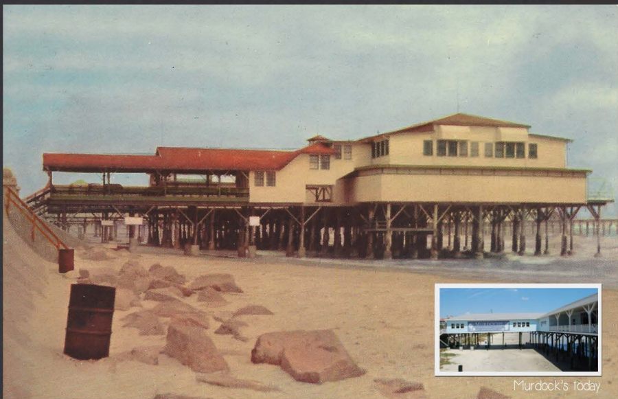
Murdock's Bath House, this structure was heavily damaged by Hurricane Carla in 1961. It has since been rebuilt and is now called Mudrock's Gift Shop.
